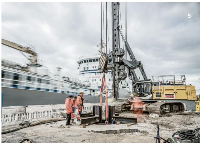
1 Trough excavation pits, A100 motorway ring, Berlin/ 2 Detail of new construction Main Collection West, construction of underground station, Stuttgart 21/ 3 Bored pile shaft, supply culvert, Kiel-Holtenau lock, © Sebastian Engels Photography, www.sebastian-engels.de/ 4 Ground freezing of protective roof, Severinstraße underground station, Cologne/ 5 Steel pipe shafts, supply culvert, Kiel-Holtenau lock, © Sebastian Engels Photography, www.sebastian-engels.de/ 6 Extension of MCT quay, Port Louis, Mauritius
