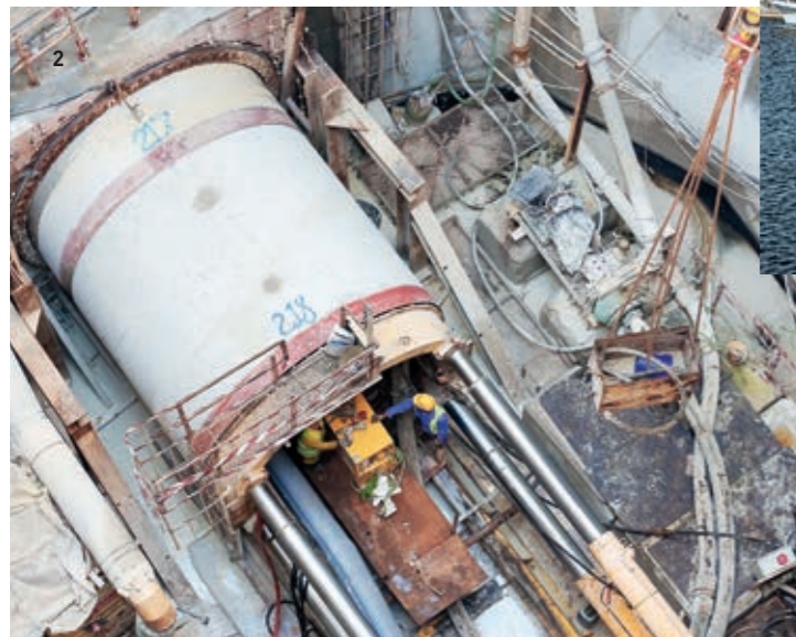
1 Subaquatic Tunnelling Söderströmstunnel, Sweden / 2 Pipe Jacking STEP, Abu Dhabi
