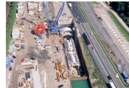
4 Mechanised Tunnelling, Jenbach H8, Austria
