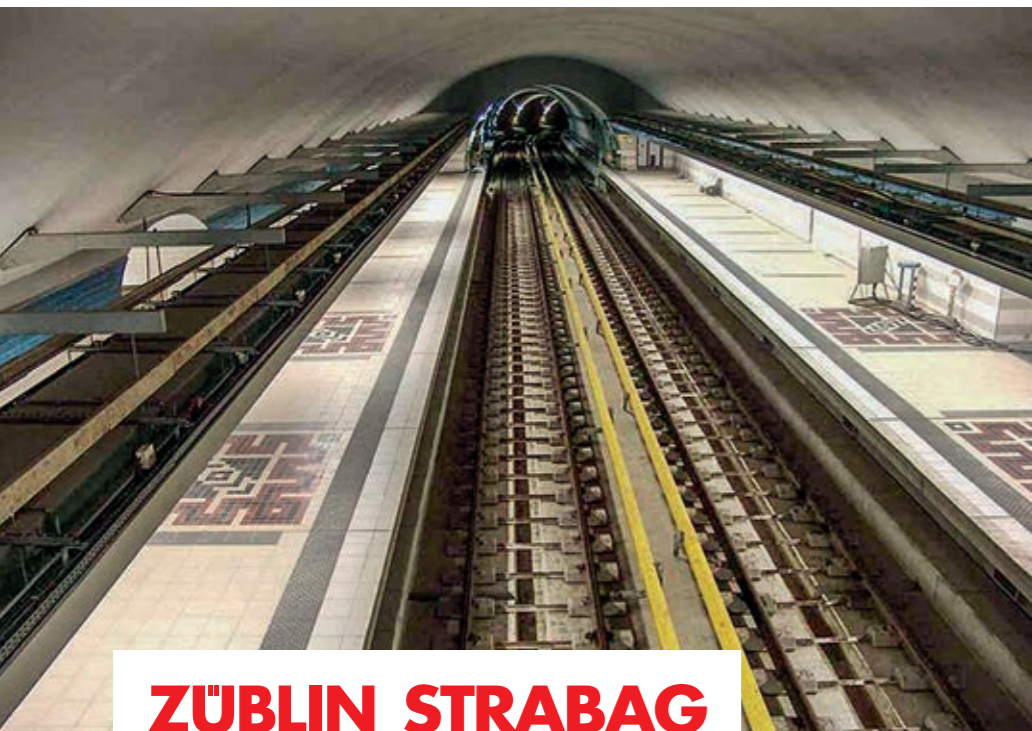
Metro Algier, Algeria
