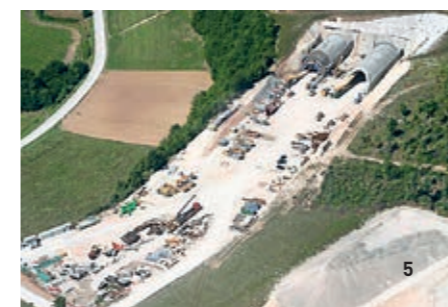
5 Concrete Tunnels/Open Pit Tunnels, Quadrilatero, Italy
