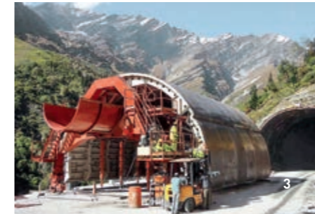
3 Conventional Tunnelling, Rohtang Pass, India
