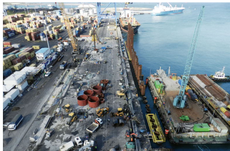
1 Hennetal Dam, Germany 2 Middle Marsyangdi HEPP, Nepal 3 Sheikh Khalifa Bridge, Abu Dhabi, UAE 4 Port Louis Container Terminal, Mauritius
